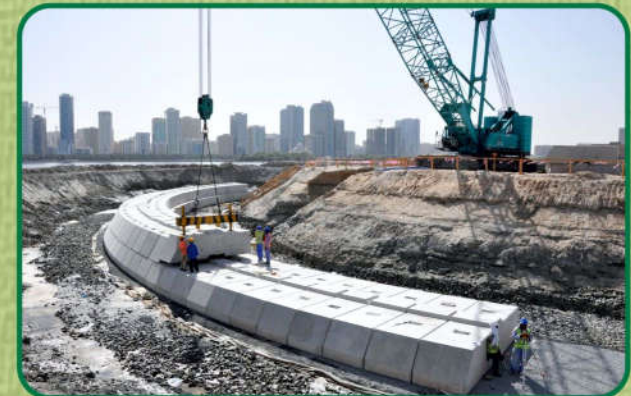
Heavy Retaining Walls
