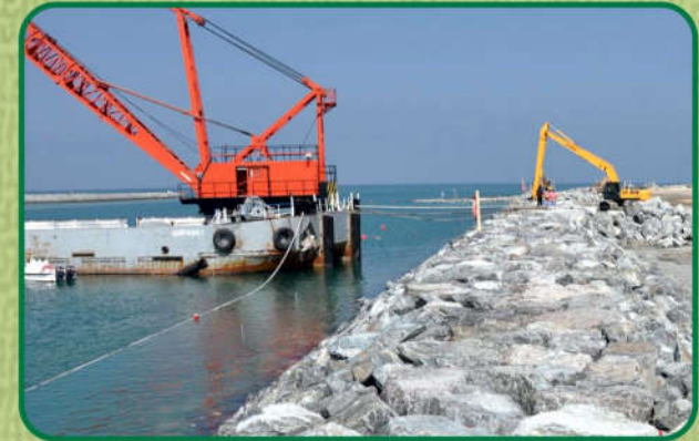
Marine Concrete Works
