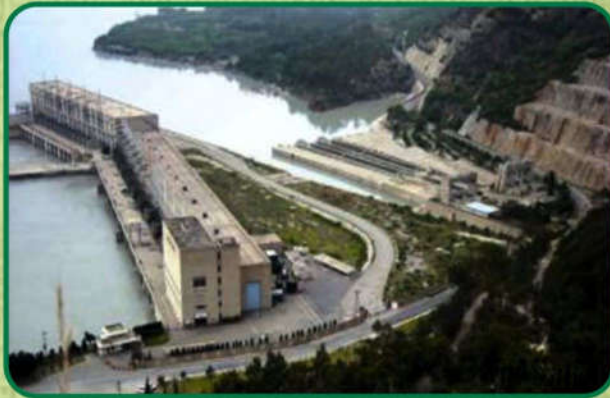
Karot Hydro Power Project
