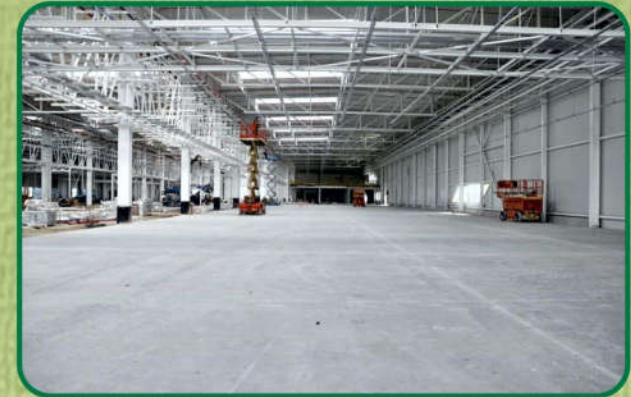
Concrete Floor for Factory
